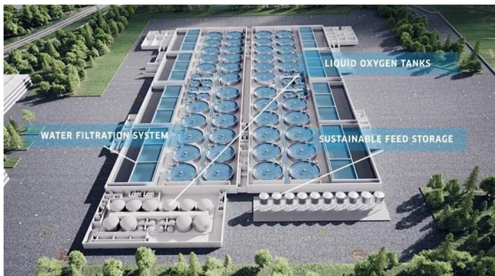
Figure 4: A model of a large RAS system
